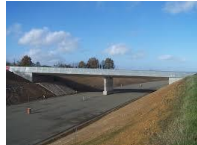
Picture of the 21.5 m long bridge
