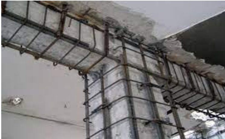
✓ Reinforced Concrete Jacketing
