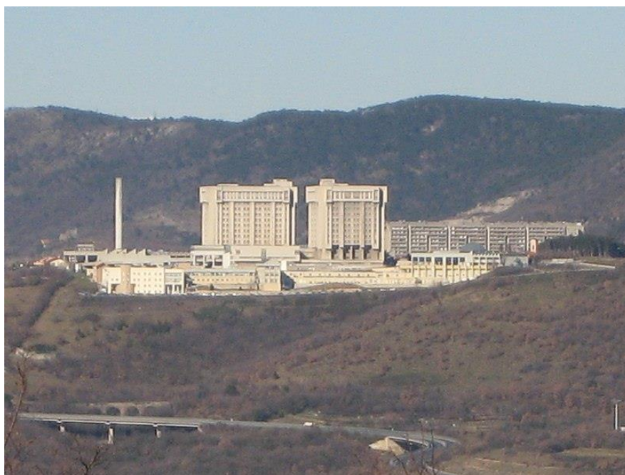
Figure 14. Cattinara hospital (source: commons.wikimedia.org)
