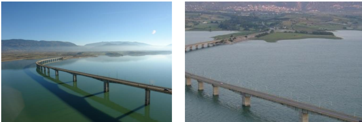
Figure 2. The Landmark Polyfytos Road Bridge.
